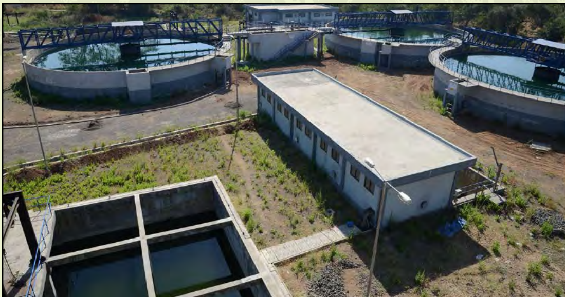
Membrane filtration plant at Bhandup Complex
